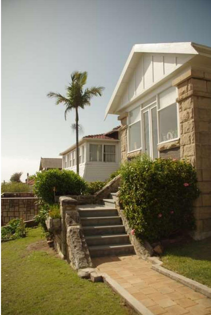
Fig.4 Enclosed front verandah showing recent new paving to stairs and also illustrating the quality of stonework employed in the verandah columns.
