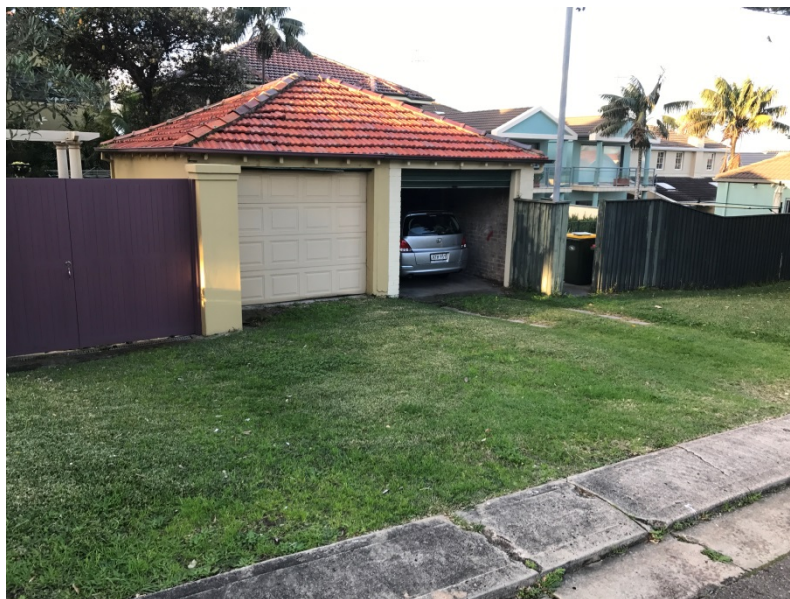
Figure 1: Existing garage on the subject site (left) and neighbouring garage (right)
