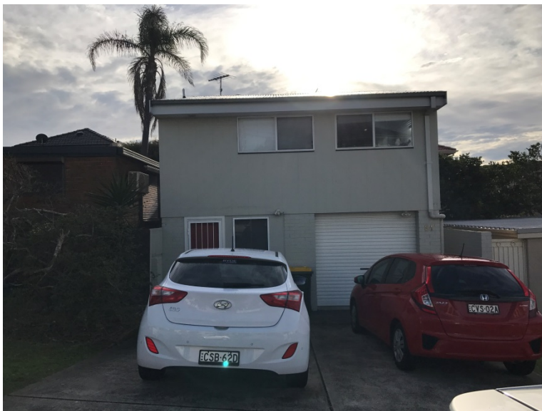
Figure 3: Garage with 2-storey dwelling component at the rear of 81 Torrington Road
