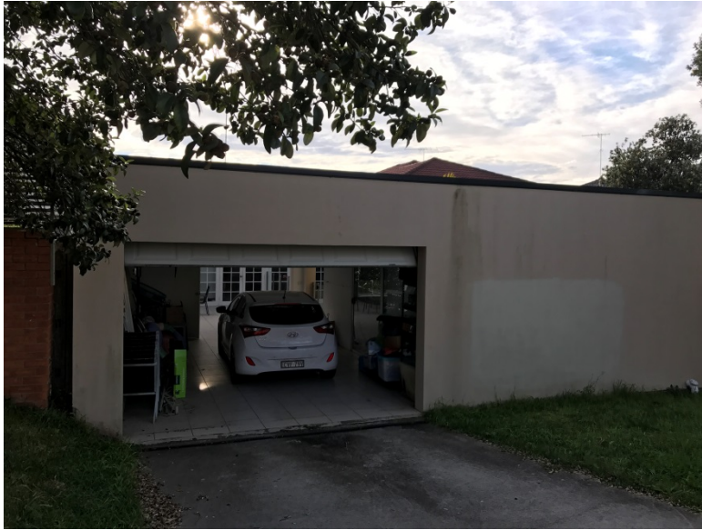
Figure 2: Garage structure at the rear of the western adjoining property
