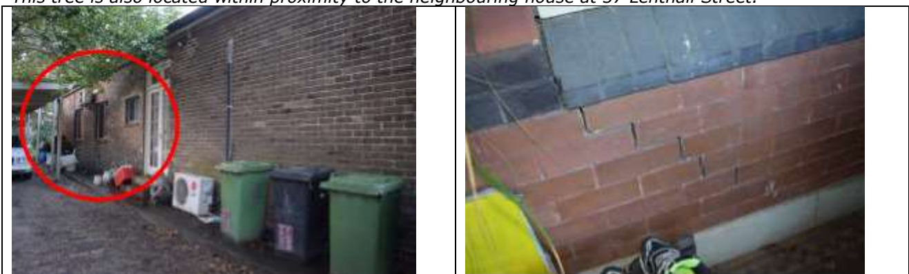
Figure 1: View looking towards the front high brick piers and wall fence, a later addition, which has a large central crack (left) and an image of the tree located in the south western corner of the site (right). This tree is also located within proximity to the neighbouring house at 37 Lenthall Street.
