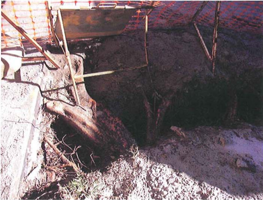
Numerous tree roots (incl. one very large root) growing under footpath and driveway
