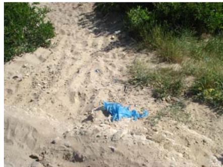
**Photo 4** Waste materials exposed by surface erosion of the landfill
