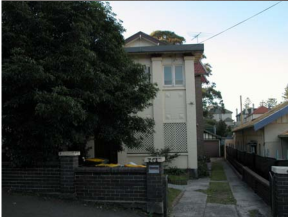
Figure 3: No. 45 Dudley Street adjoining the site to the west.
