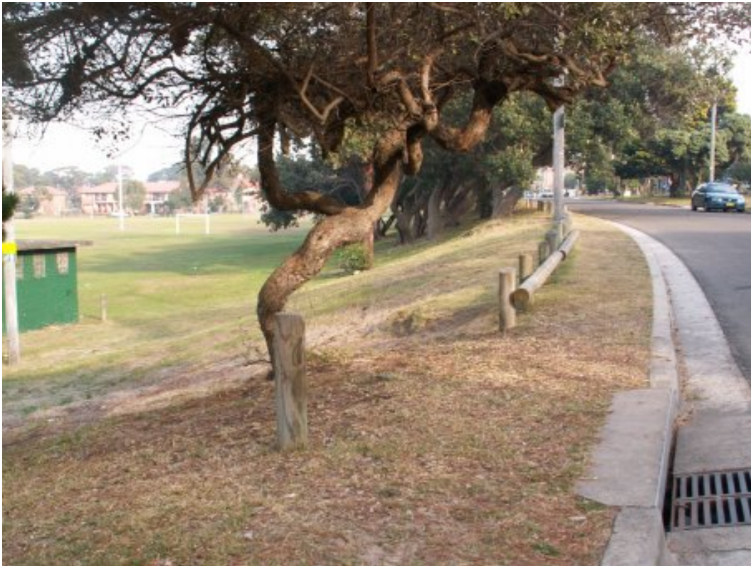
Image 2 View of the embankment behind the amenities building.
